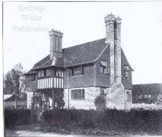
“MOORHATCH” HORSSELL A handsome example of 20th-century style, with occasional red brick and a roof of stone and slate tiles. The houses are built glass and all the windows, including the front windows, are made with hand-made glass.
