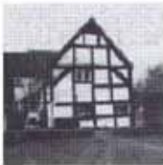
Whapshott Farm – rear view.
